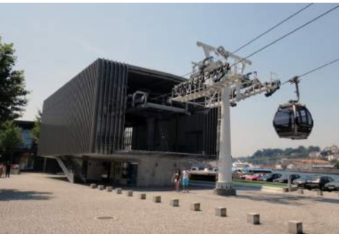
Small station footprints allow gondola systems to be built in land-constrained areas.
