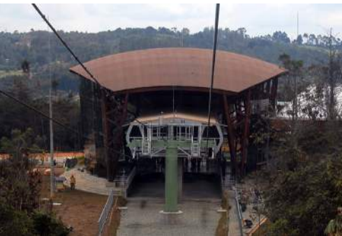
Medellin's Line L stations are designed with a wrap concept which improves aesthetics but remains cost effective.
